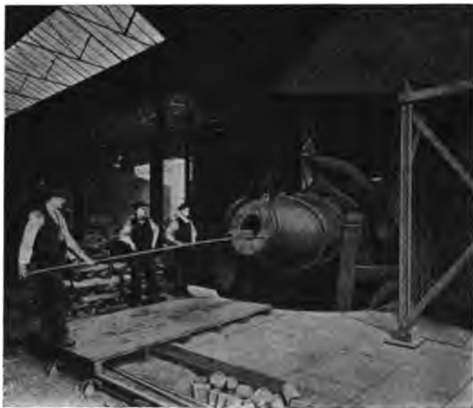
FIG. 232.—Stock Converter. Charging Position.
